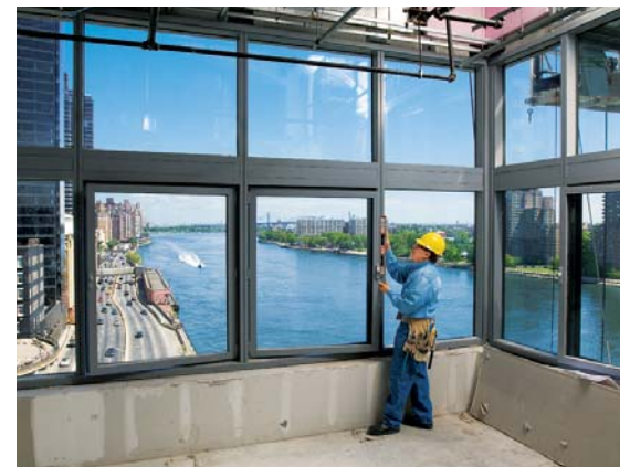
△ New patient rooms, currently under construction, will overlook the East River.
